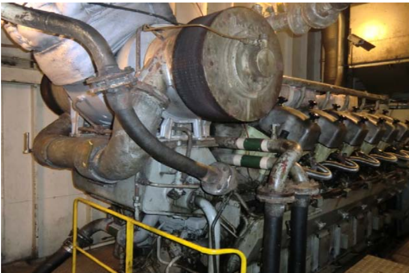
Before Retrofit: NR26/R
