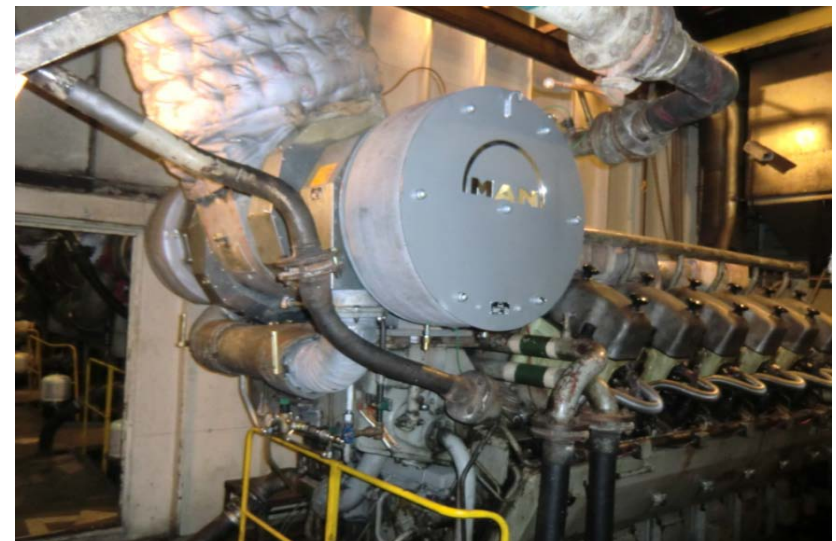
After Retrofit: TCR20-4
